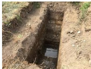
Trial pit / excavation
