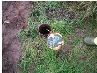
Standpipe in backfill
