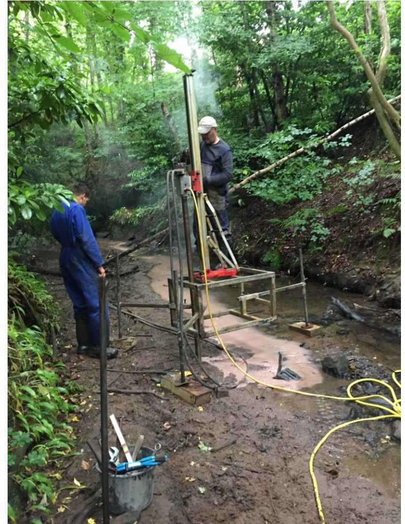
Investigation to install drive points in Burn
