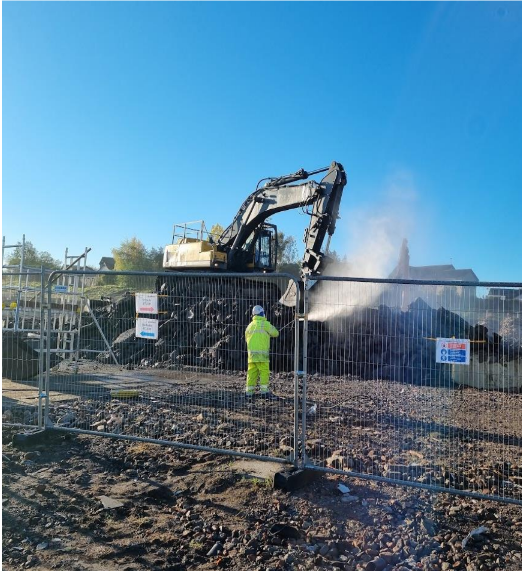
Asbestos dust suppression measures
